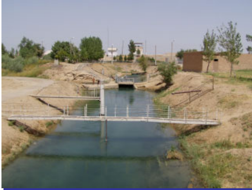
Figure 12. Hydro junction from Uchkzyl water reservoir and an Uzbek army lookout in Kattakum, Uzbekistan, August 2002. Photo by K. Toderich.
